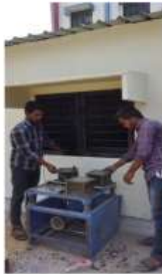
Fig 3.7.3 Vibrating the moulds
